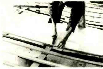
FIG. 16—AFTER STAPLING ONE EDGE, keep the screen taut and staple the point directly across from the first.
