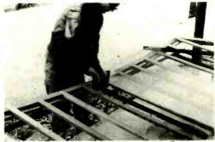
FIG. 17—PULL THE ENDS tight enough to keep the screen straight from center to edge. But, don't pull too tight—the screen may pucker in the middle.
