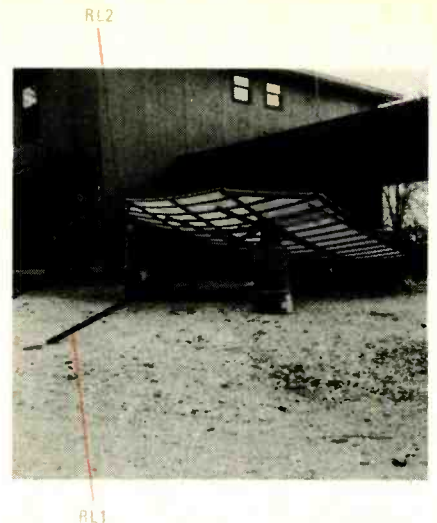
FIG. 21—THE TOP END OF THE ANTENNA is raised three to four feet off the ground so rear legs RL1 and RL2 can be attached. Put small blocks under the lower end to protect the corner adjustment bolts.
